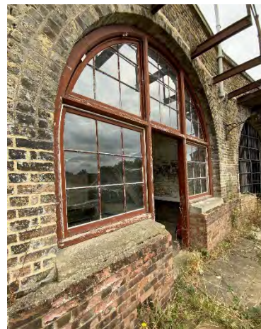
Figure 108 Exterior of Room Number 5
