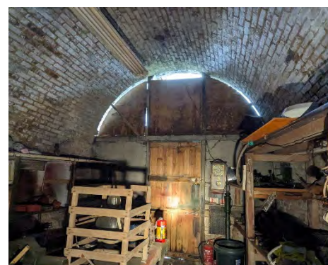
Figure 93 Interior of Casemate B15
