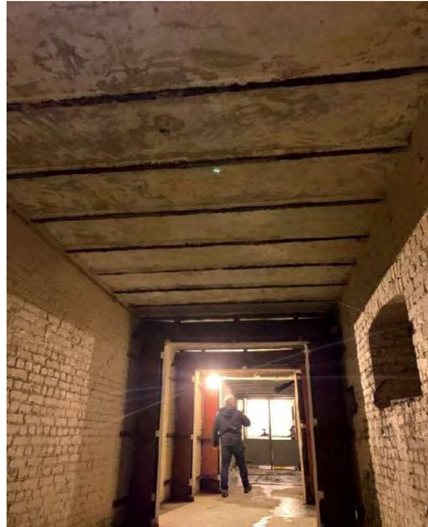
Figure 150 Narrower north end of roof
