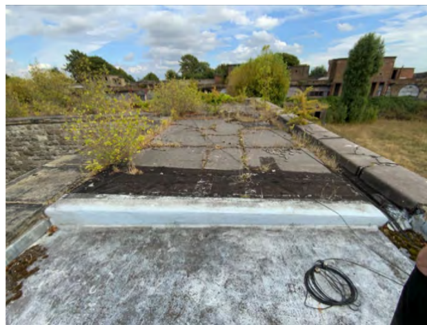
Figure 57 Roof – North Range
