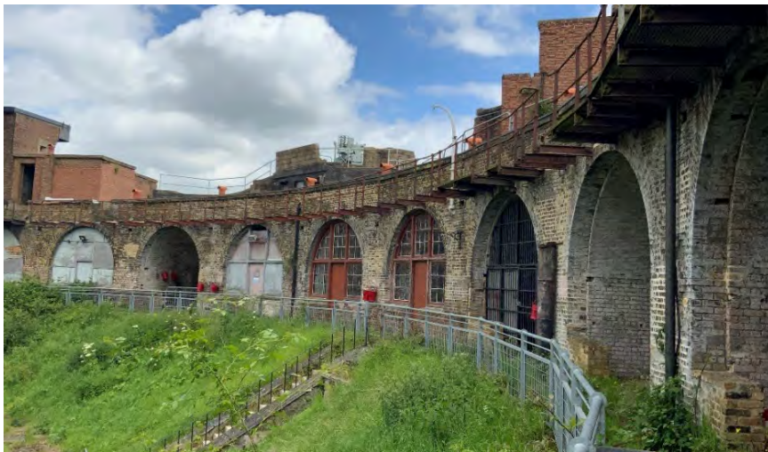
Figure 127 Access routes to casemates
