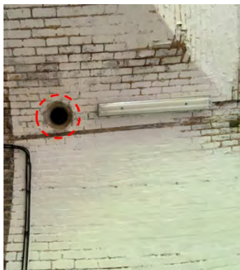
Figure 138 Ventilation of lining could utilise the existing flues originally provided for purging of smoke within the Casemates from firing the guns
