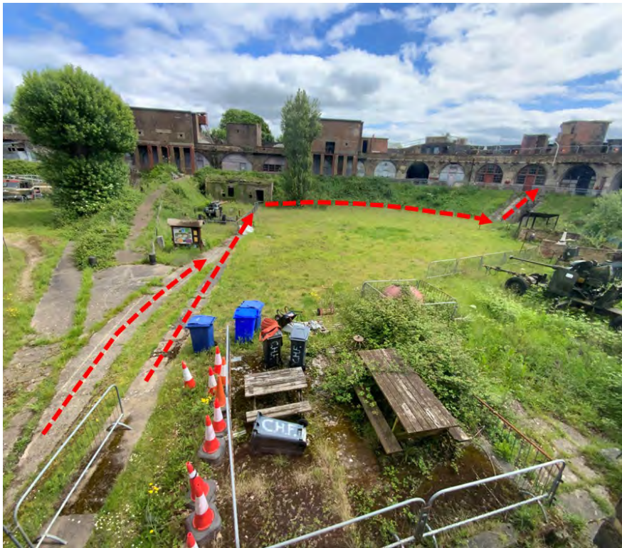
Figure 125 The Parade Ground has existing concrete paths around the perimeter leading to ST/03
