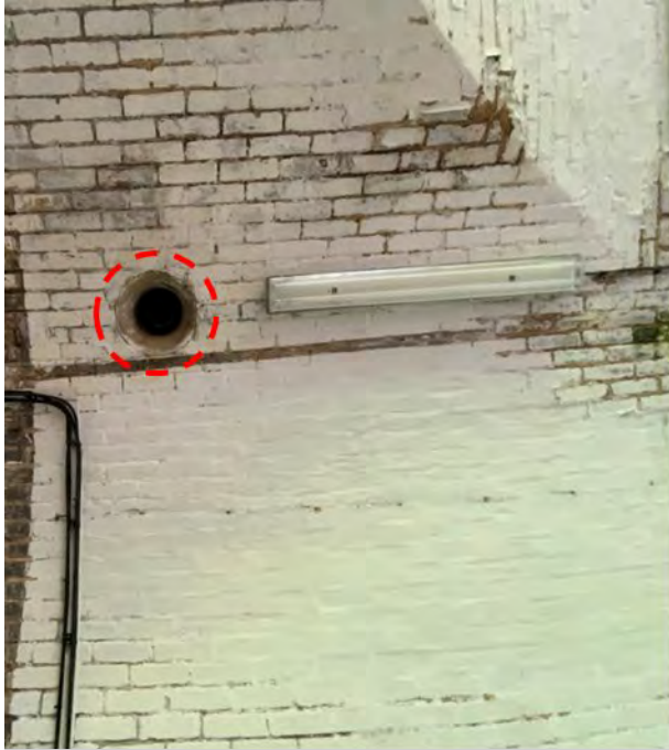
Figure 146 Ventilation of spaces could utilise the existing flues originally provided for fireplaces and purging of smoke within the Casemates from firing the guns
