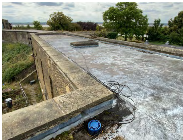
Figure 58 Roof – West Range
