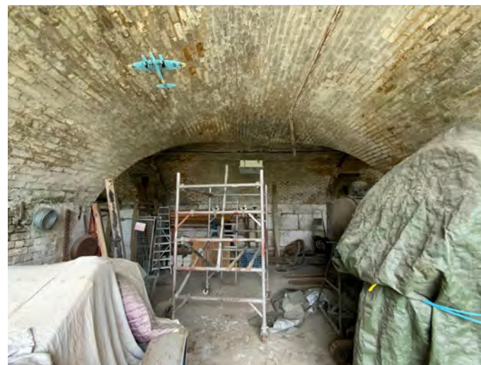
Figure 103 Interior of Room Number 3
