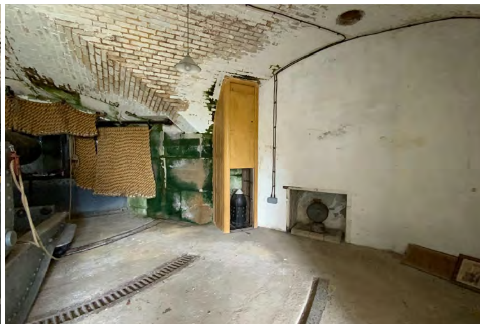
Figure 113 Room Number 6 (2) view of the former shell lift
