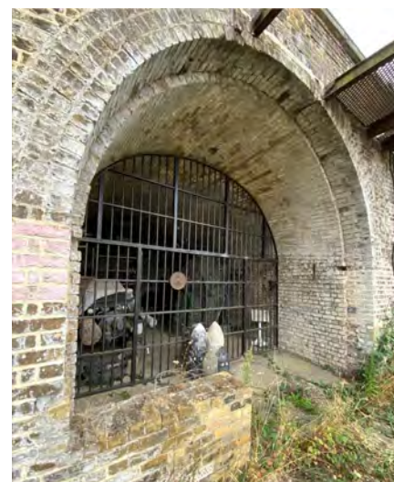
Figure 104 Exterior of Room Number 3
