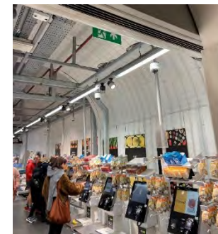
Figure 140 (Above) Examples of lining to brick railway arches using corrugated plastic sheet lining (London Bridge Station)
