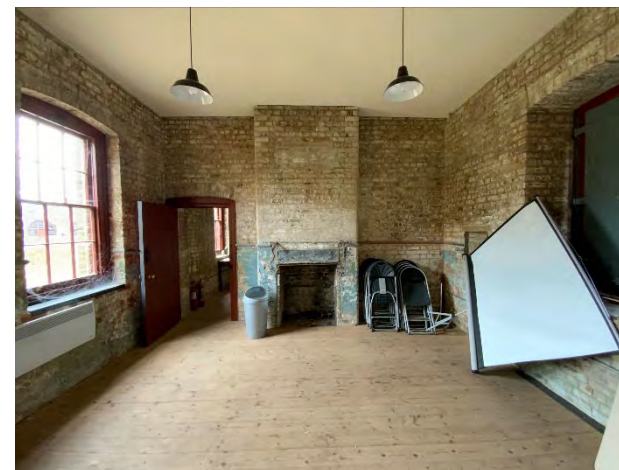
Figure 53 View north into room number 1/06
