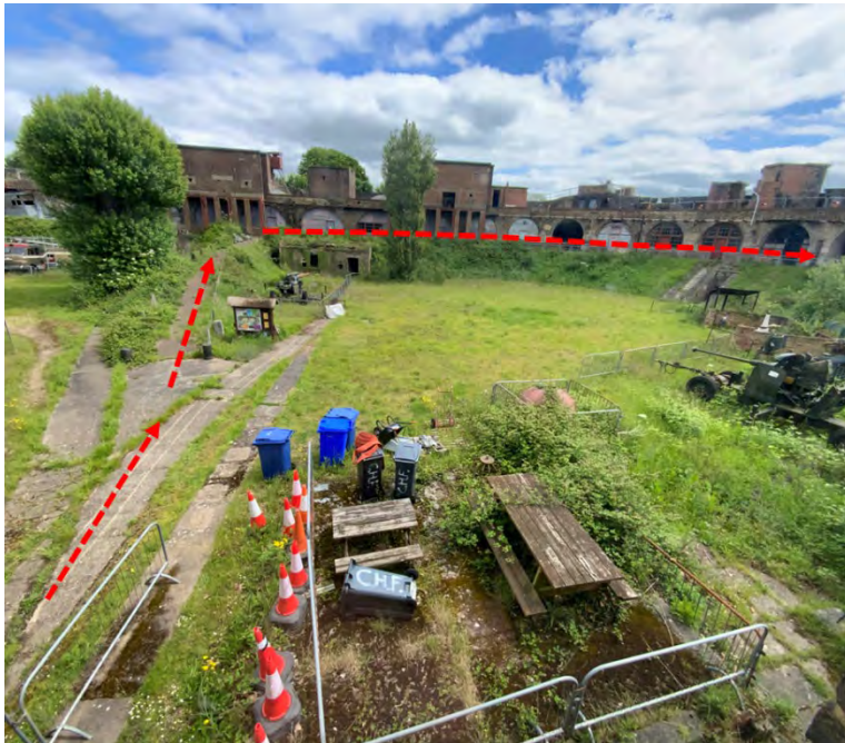
Figure 123 The East Ramp provides access to the Casemates Walkway at the upper level
