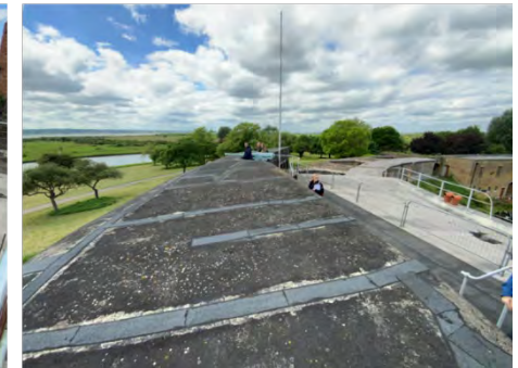
Figure 119 View west across the roof
