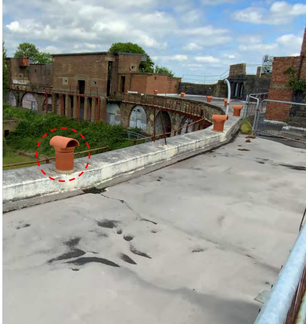
Figure 147 Exterior existing flues
