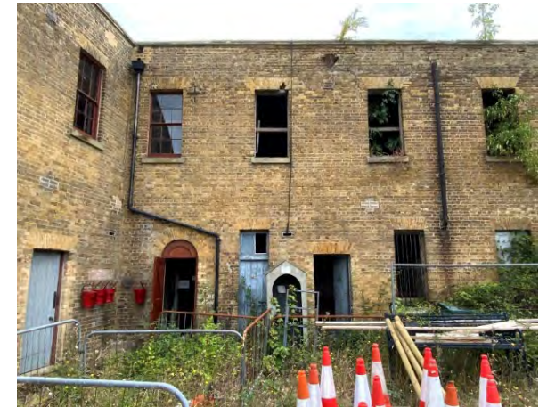
Figure 60 View of the internal south elevation
