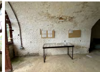
Figure 110 Interior of Room 6 (looking east)
