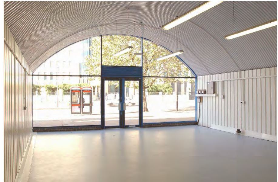
Figure 136 Example of aluminum glazed screen to a vaulted space, with minimal sightlines to the framing and maximising admittance of daylight to produce a streamlined aesthetic with good amenity. The Casemates arches were originally open, which would be perpetuated by the use of minimal framing and larger expanses of glass.
