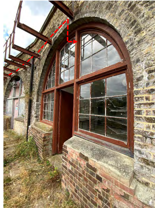
Figure 134 Services are provided via the existing disused external walkway running above the entrances of each of the Casemates. The entry point into the spaces is via the entrance screens, either by carefully removing a section of glazing in the existing glazed screens or via purpose-made entry points within new screens
