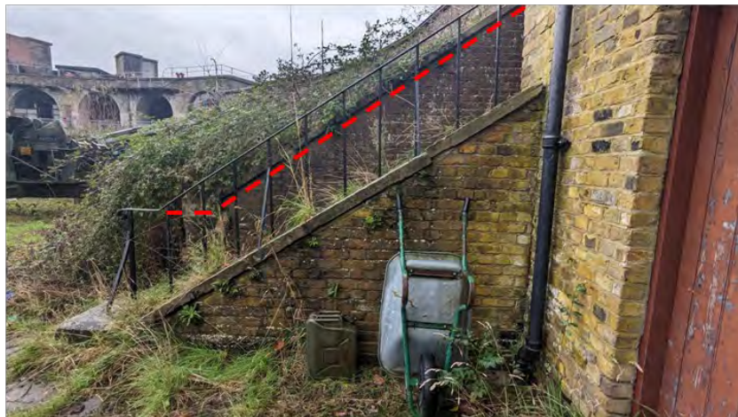
Figure 73 ST/01 a continuous handrail provided to the south side of the stair in addition to the existing, improving accessibility
