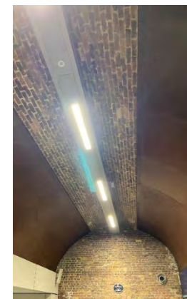
Figure 139 Examples of lining to brick railway arches using corrugated plastic sheet lining
