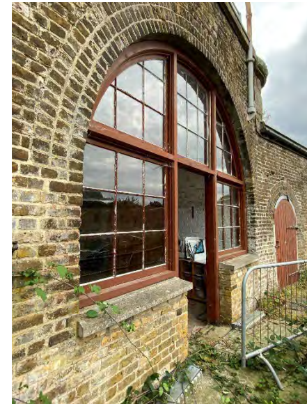
Figure 99 Exterior of Unit Number 1
