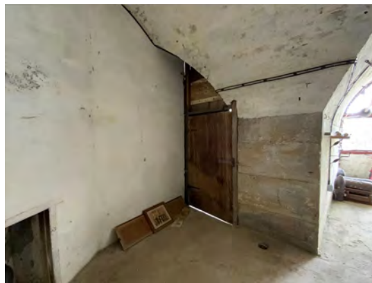
Figure 115 Room Number 6 (4) view north towards the entrance of the casemate
