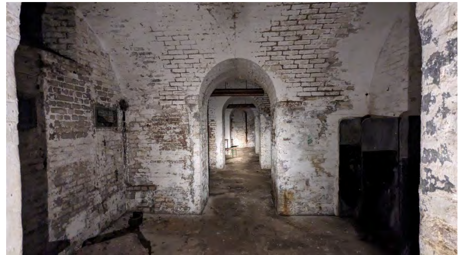
Figure 3 View of the tunnels, taken during an early site visit
