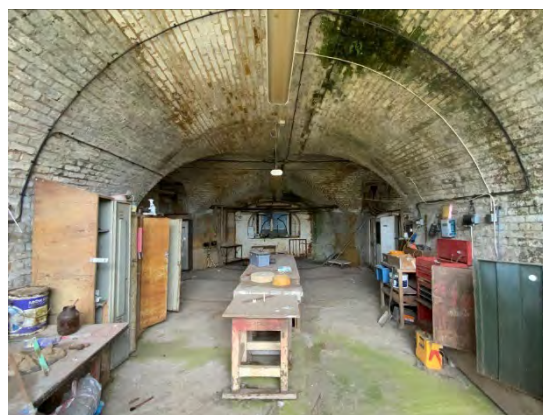
Figure 106 Interior of Room Number 4
