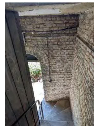
Figure 34 Access to the upper floors of the Gatehouse
