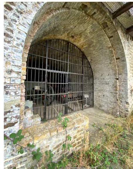
Figure 102 Exterior of Room Number 2
