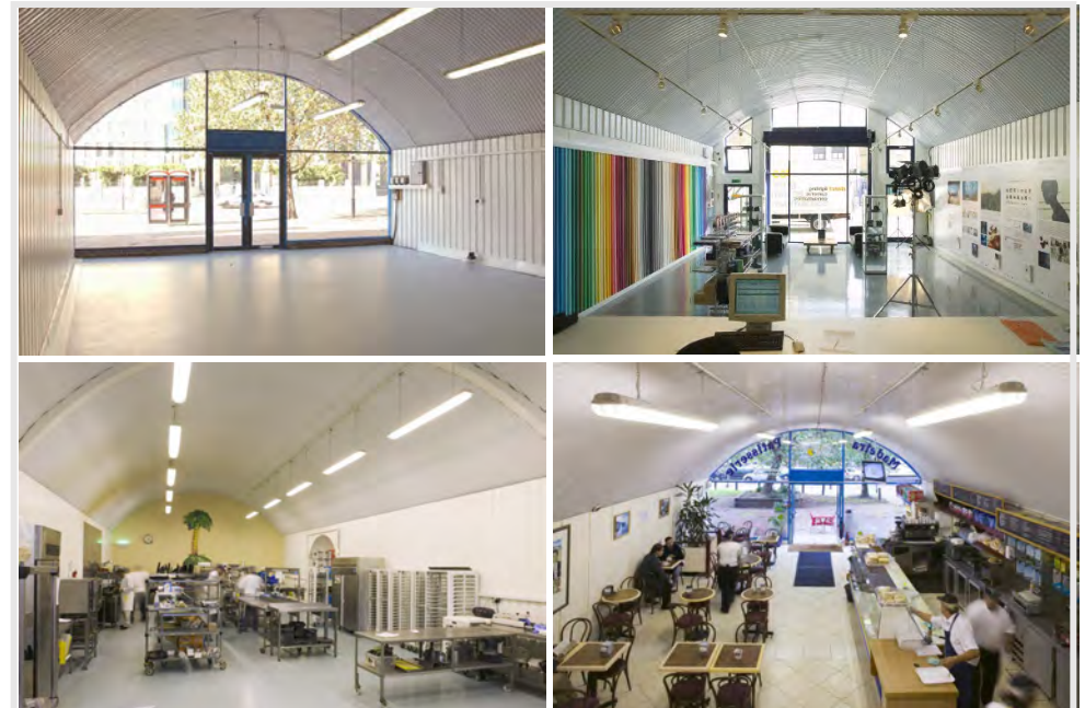
Figure 139 Examples of lining to brick railway arches using corrugated plastic sheet lining
