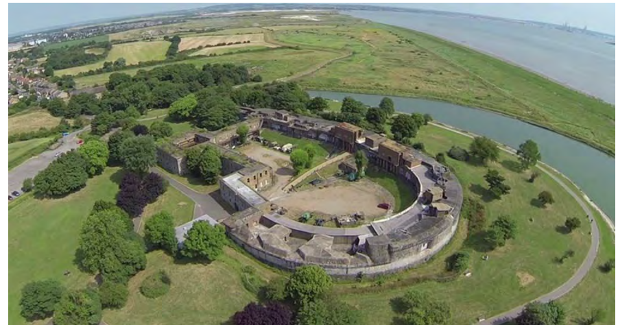
Figure 10 Coalhouse Fort from the air
