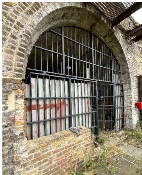
Figure 105 Exterior of Room Number 4
