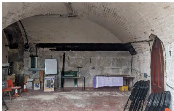
Figure 92 Interior of Casemate B09
