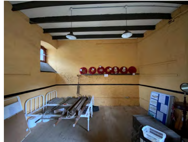
Figure 41 View north into room Number G/05
