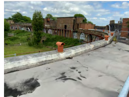
Figure 118 View north east across the roof
