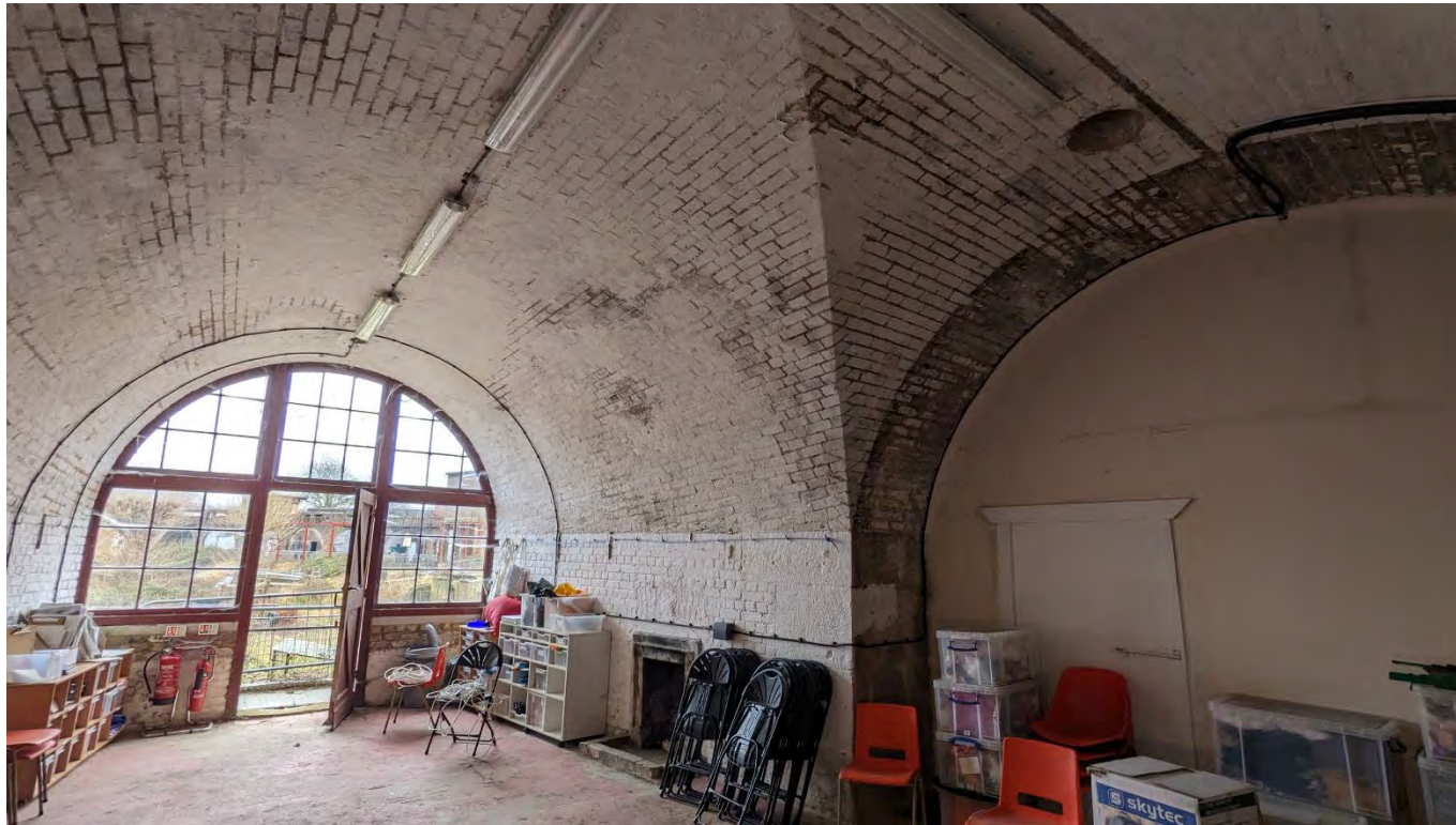
Figure 148 Internal view of the casemate
