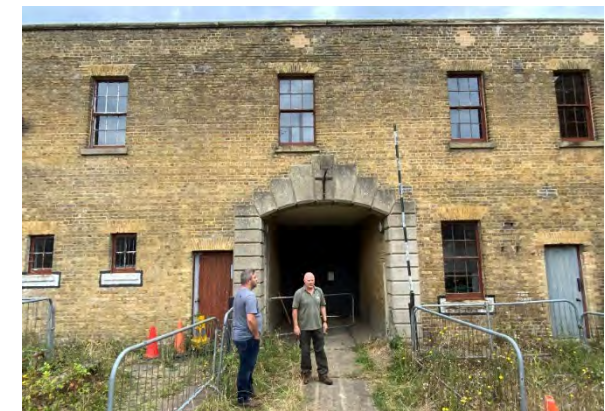
Figure 61 View of the internal east elevation
