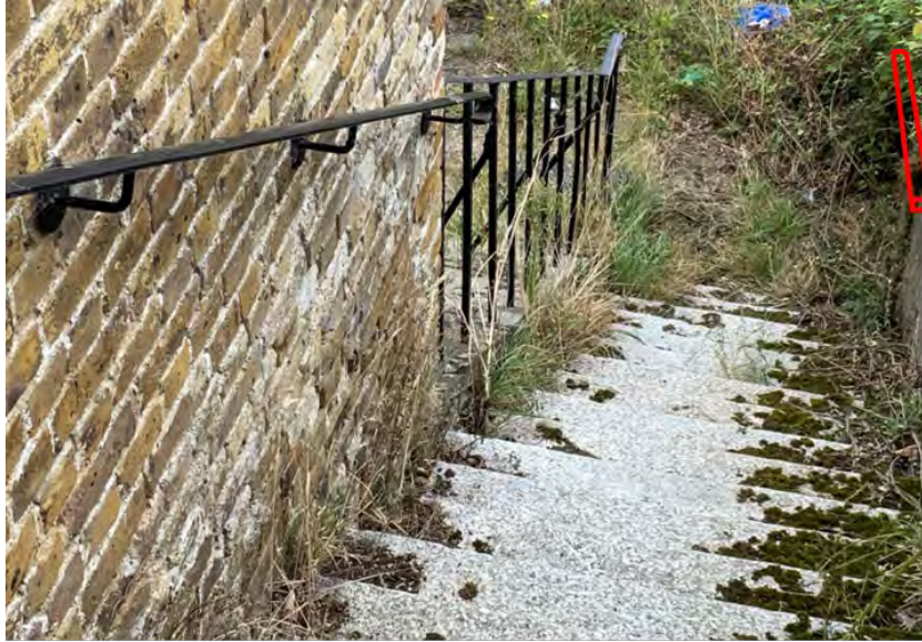
Figure 72 Vegetation on ST/01 will be cleared
