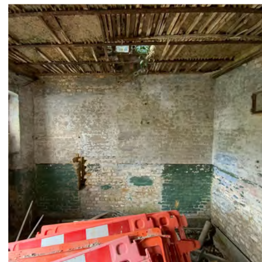
Figure 45 View into room G/06 (3)
