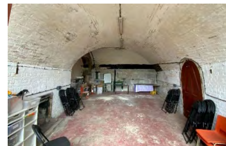
Figure 100 Interior Unit Number 1
