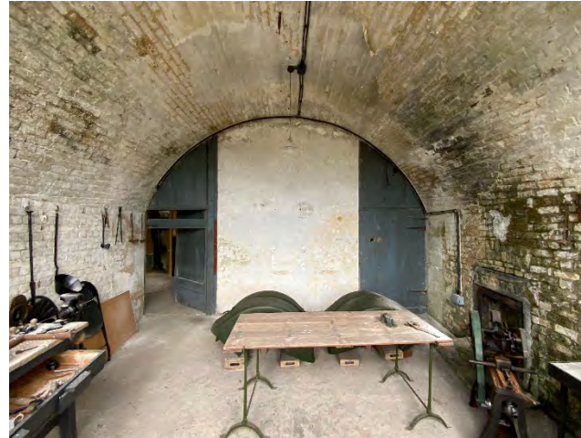
Figure 107 Interior of Room Number 5
