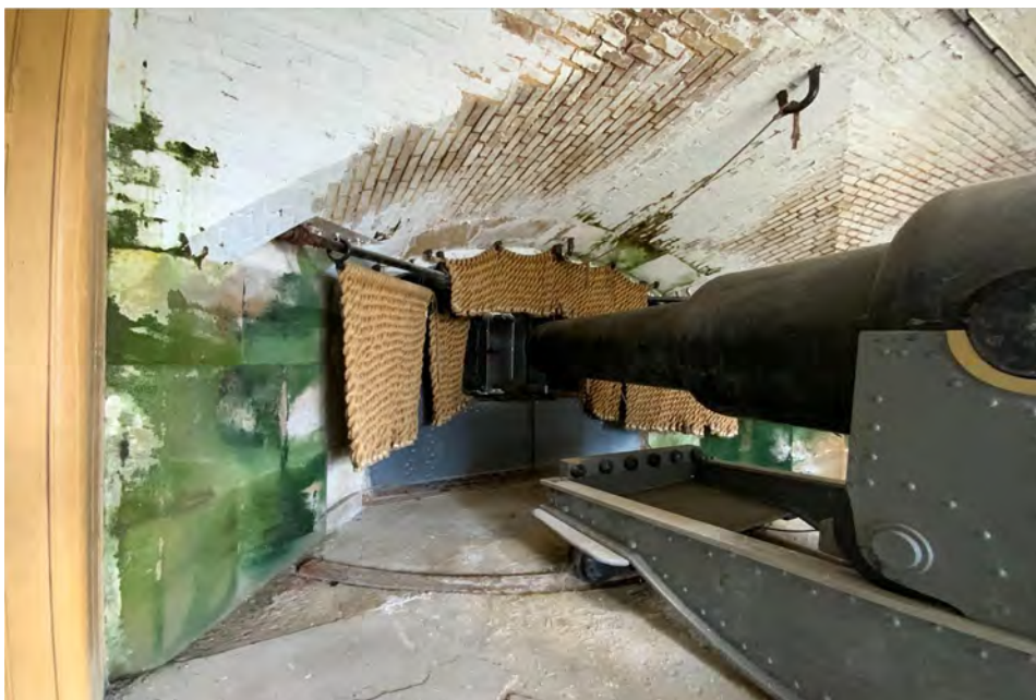
Figure 112 Room Number 6 (1) looking south towards the gun port
