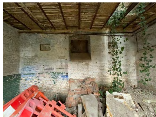
Figure 43 View into room G/06 (1)
