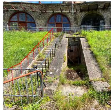
Figure 121 ST/03 vegetation will be cleared, and a continuous handrail provided to the east side of the stair in addition to the existing, improving accessibility. The existing balustrade may need to be raised and infilled between balusters, dependent on building regulations
